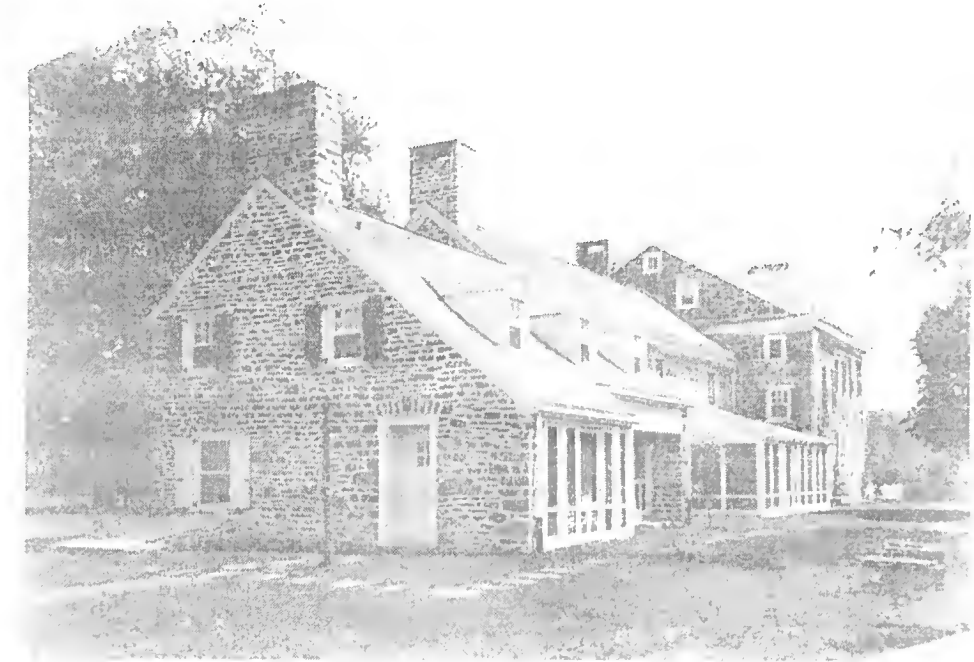
Figure 34 North and West Facades of Manor House, looking southeast, c. 1930
